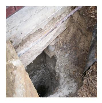
ote the concrete cylinders adjacent to the shaft, these are "pressed piles" or what we prefer to call "pushed cylinders".
